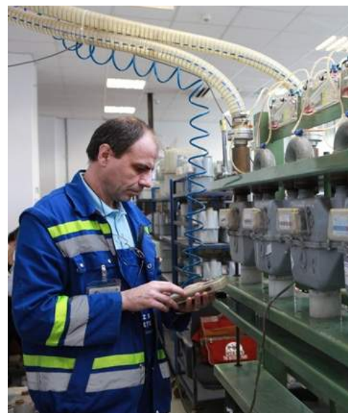
Image courtesy of GDF SUEZ Energy Romania.
